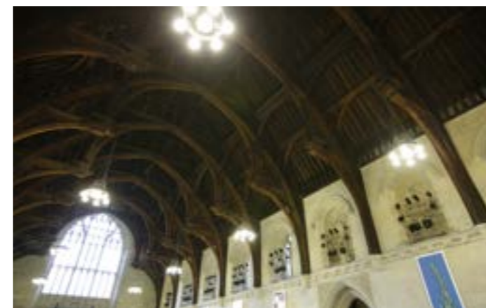
The hammer-beam roof of Westminster Hall in the Palace of Westminster
